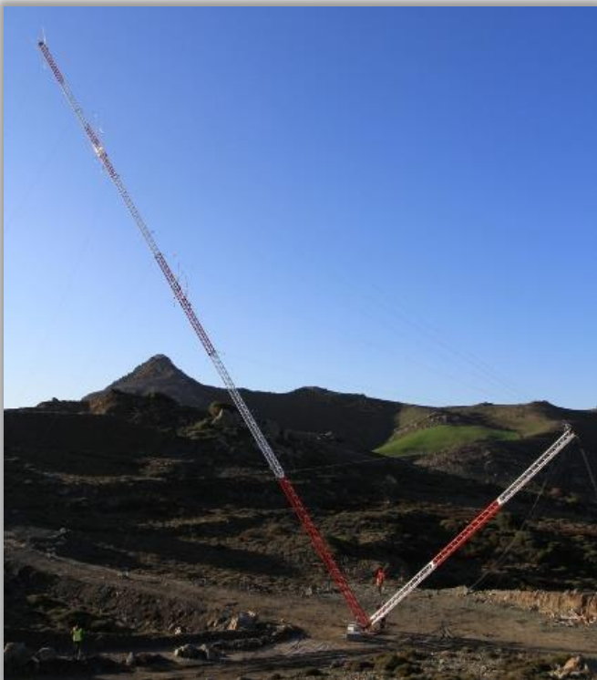
Tilt up Lattice tower during erection
