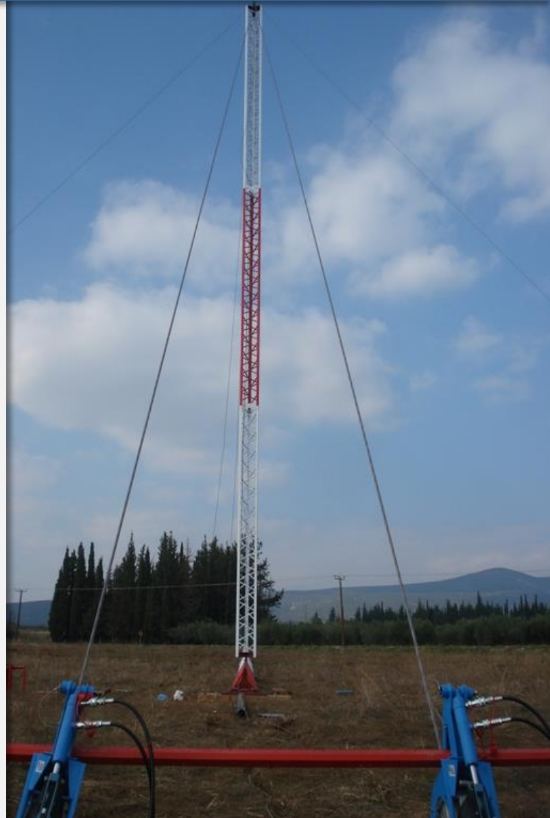
Tilt up erection with tirsors
